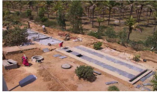
Fig 11. A DEWATS after completion
