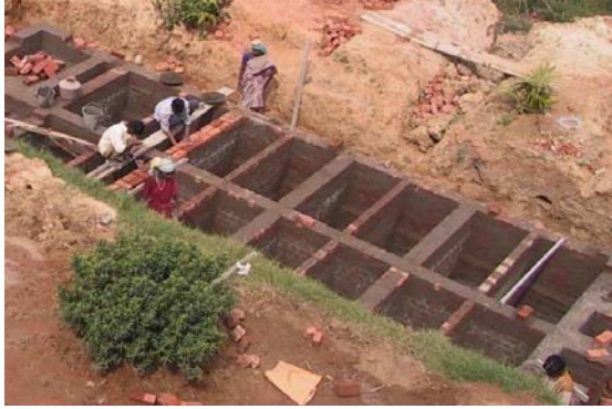
Fig 10. A DEWATS under construction
