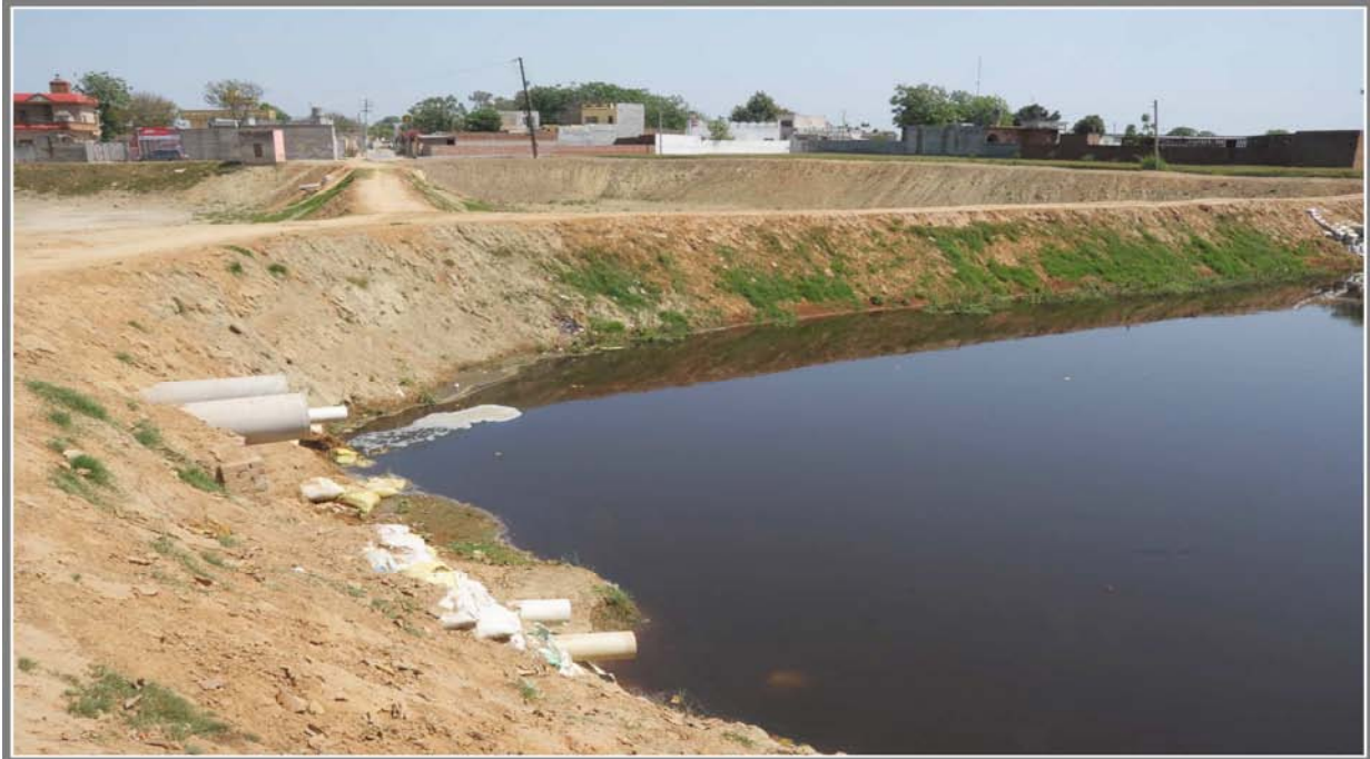
Fig 2.1. A Stabilisation Pond System in Dewatwal village (Ludhiana District, Punjab)
