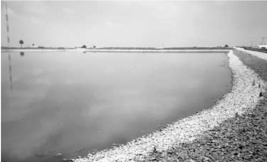
Fig - 4 Use of boulders to check erosion of embankment
